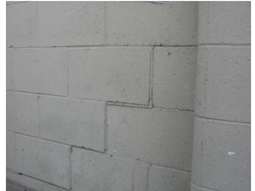
Typical "Stair Step" Cracking
