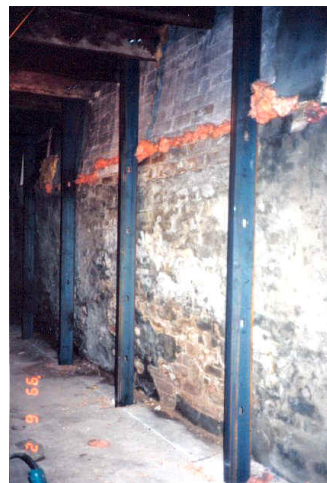
Some examples of bracing using steel members
