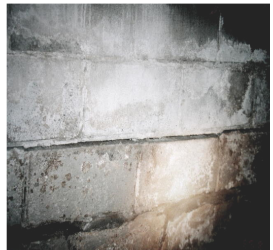
Example of a horizontal crack
