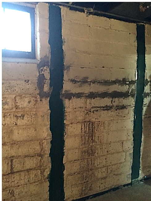
Example of installed carbon fiber strap system
