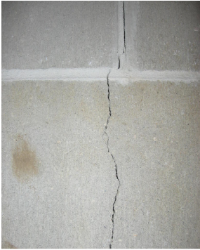
Typical vertical cracking
