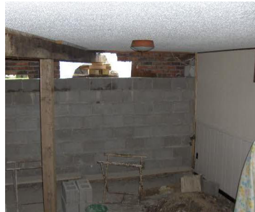
One basement wall undergoing complete replacement
