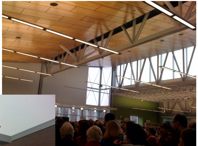
Photo right showing exposed steel trusses
