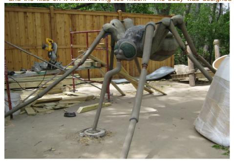
together to give shape to the body and to provide the stiffness needed. At the suggestion of Themescapes, the body was re-analyzed using a steel plate down the middle of the body, with additional plates welded out of it to create the shape of the mosquito body.
