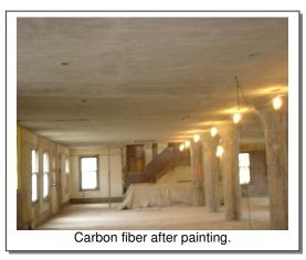
had been around for centuries, it had not been used in conjunction with steel rebar in this fashion, which uses draped steel rebar on continuous thin spans in all directions, a 4-way slab as it was later known as. C.A.P. Turner is also the same engineer that designed the Duluth Lift Bridge and other "mushroom" slab buildings in the Midwest.
